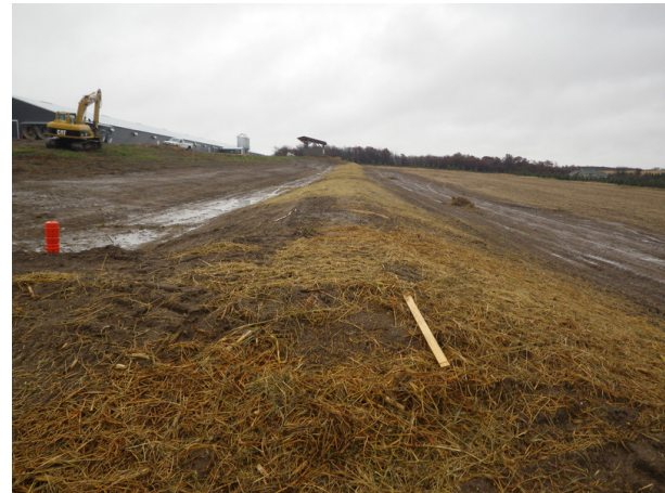
Water and sediment control basin.
