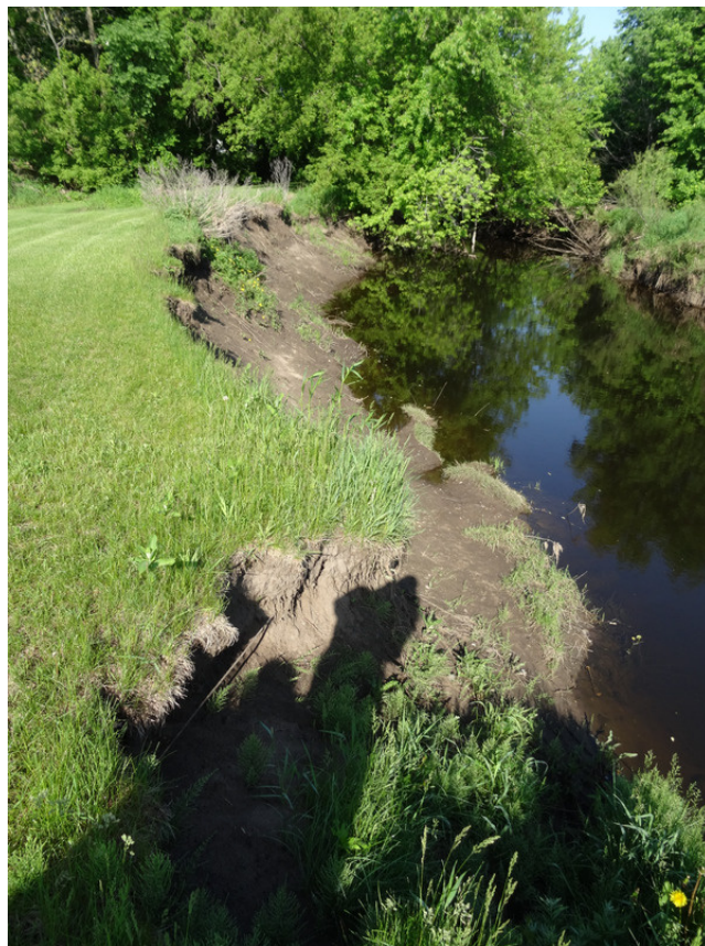
River shoreline without any natural buffer and has been mowed right to the stream bank. Stream bank erosion issues are a result.
