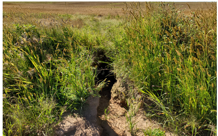
Gully erosion in Benton County.
