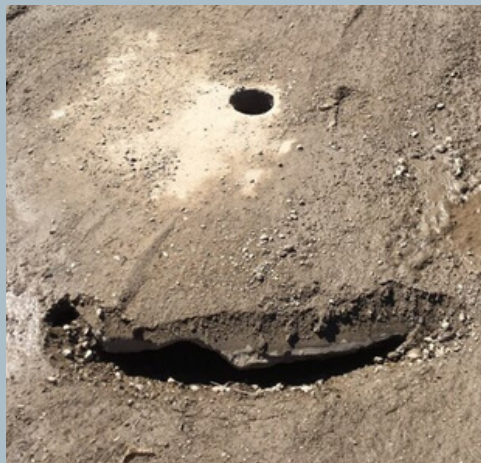
50' deep dug well sealed in 2019
