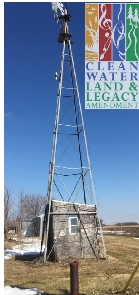
37' deep dug well sealed in 2019
