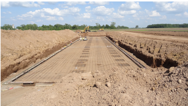
Pouring a concrete floor of a manure pit
