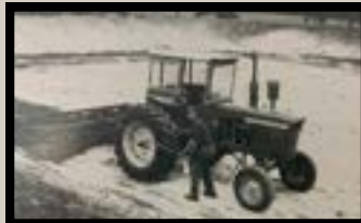
Bentonite added to the surface of the holding pit.
