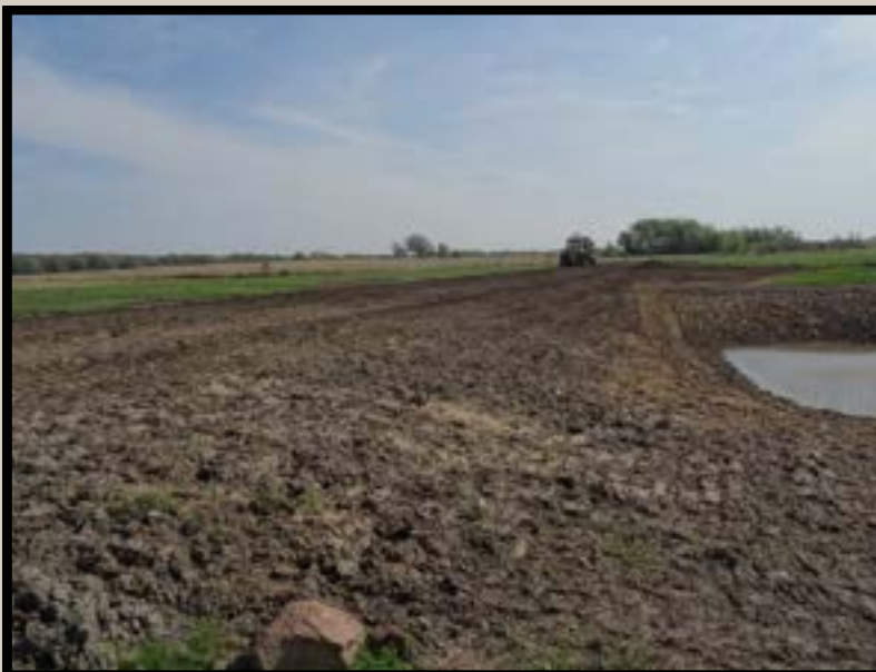
Fish barrier construction.
