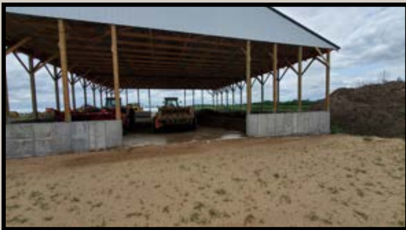
Covered stacking slab.
