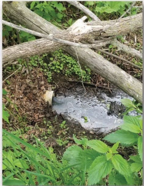
Above: Outlet Pipe Drainage
