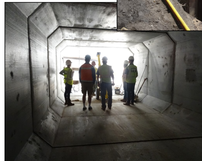
Left: View from inside the installed box culverts
