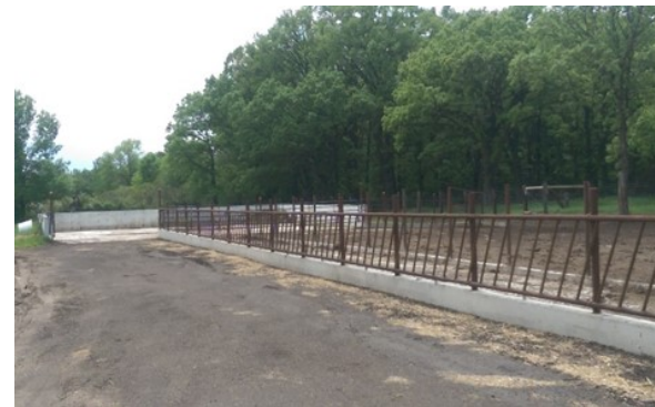
Left: Manure stacking slab and scrape lanes for beef operations.
