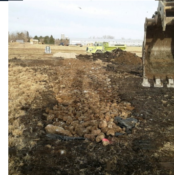
Right: Crushed rock and gravel installed
