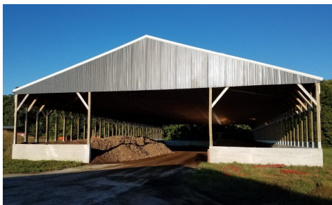
Left: Roofed-manure stacking slab for both broiler barns.
