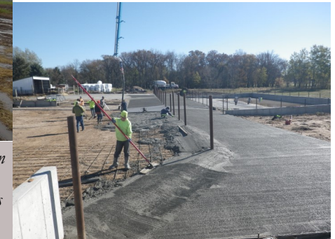
Pictured above: A water & sediment control basin as part of a cropland erosion control project. Pictured right: A beef feedlot project in the process of pouring and shaping a diversion.
