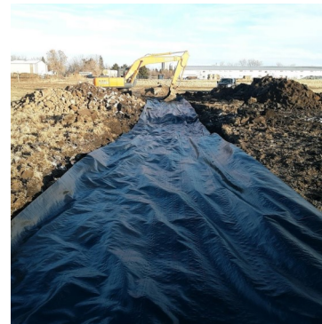
Left: Geotextile in place
