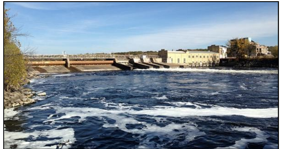
Above: Sartell Dam and powerhouse
