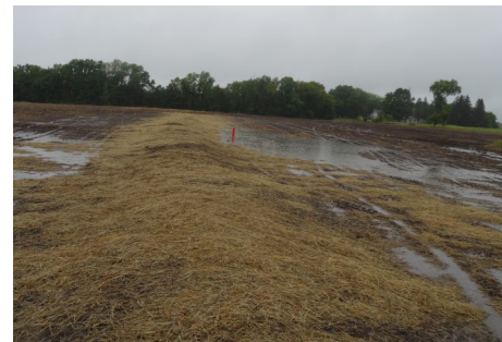
Pictured above: A water & sediment control basin as part of a cropland erosion control project. Pictured right: A beef feedlot project in the process of pouring and shaping a diversion.
