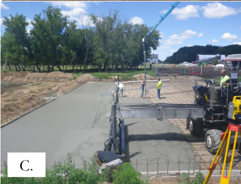
A. Stacking slab/compost facility completed for a chicken barn B. Installing and covering the GCL liner at a dairy farm C. Pouring the settling basin and stacking slab for a beef farm D. Covered stacking slab and feedlot for a beef farm
